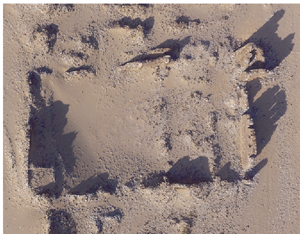
Рисунок 2. Общий вид Здания 3. Снимок с квадрокоптера И. Шкрибляк Figure 2. Overview of the Building 3. Picture from the drone was taken by I. Shkribliak
